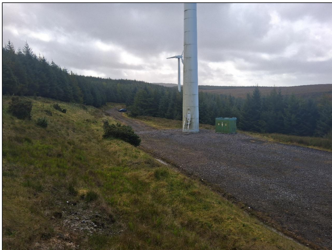
Plate 2-16 Proposed turbine 8 area - existing turbine and hardstand
